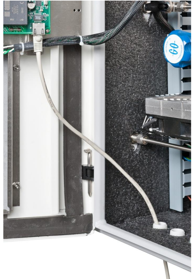
Ethernet cable installation
