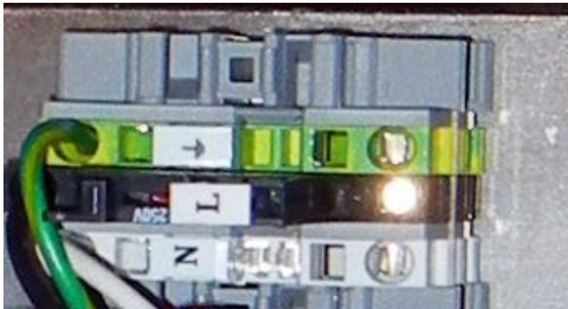
Figure (C.1)- Power Terminal Blocks, AC Version
